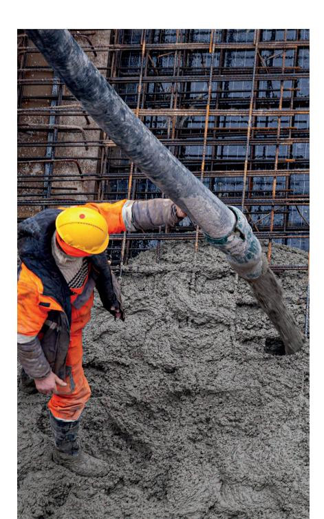
The foundation is executed with a foundation slab on a combination of piles and buried walls drilled and excavated continuously and concreted by pumping.
